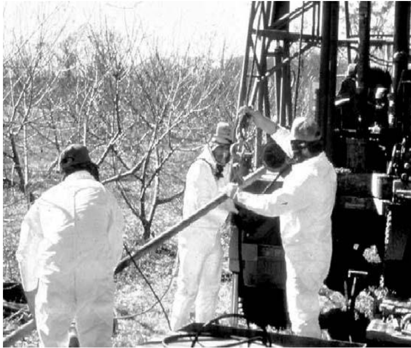
(c) Workers wearing protective clothing with supplied air respirators (SAR).
